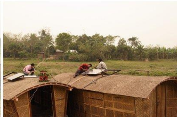
Installation of solar panels onto boats selected for educational use
