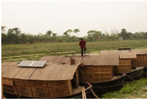
Installation of solar panels onto boats selected for educational use
