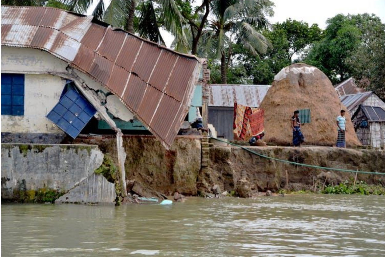
The only primary school in Singpur village is no longer safe to use due to riverbank erosion. Sonja Ayeb-Karlsson, Author provided
